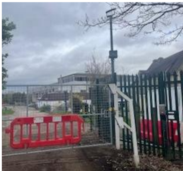
S-022 A: View of Devonport house looking north off Durley Park
